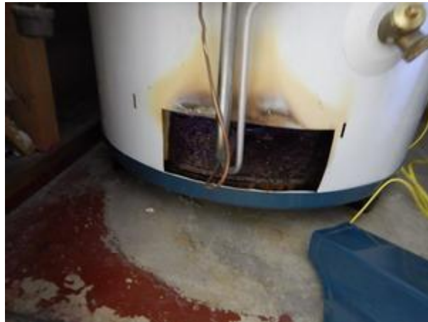
scorching at burner compartment opening
