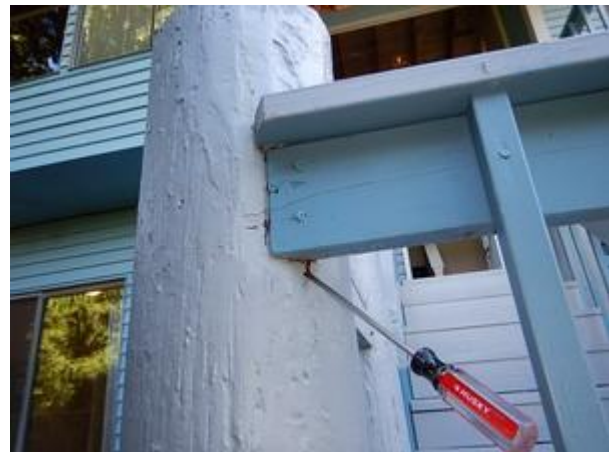
decay noted in all of the peeler poles
