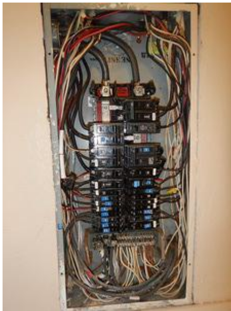
26 General Electric split-bus circuit breaker panel 27
