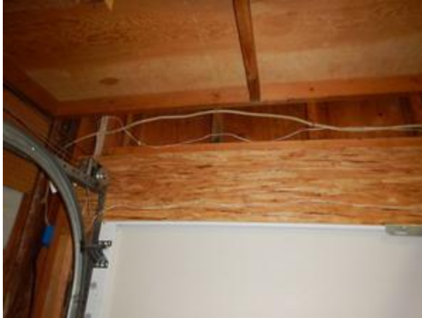
micro-lam header over garage doors
