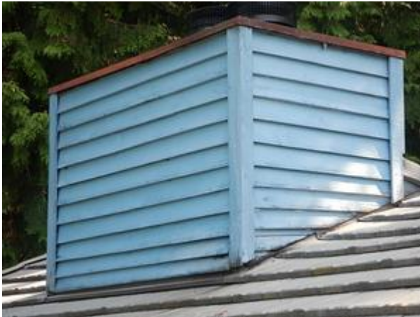
wood lap siding is overdue to be painted
