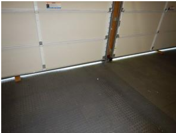
resistance activated safety stops not functional
