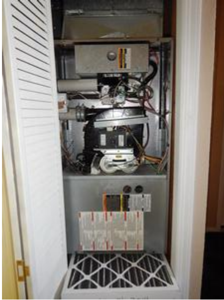
Bryant/Carrier induced-draft gas-fired furnace 3 inch clearance to combustibles not achieved
