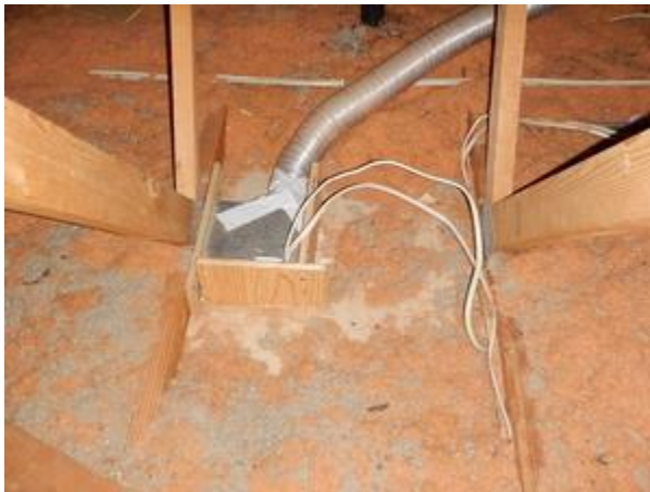
disturbed/missing insulation at retrofit fans
