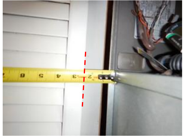
Bryant/Carrier induced-draft gas-fired furnace 3 inch clearance to combustibles not achieved
