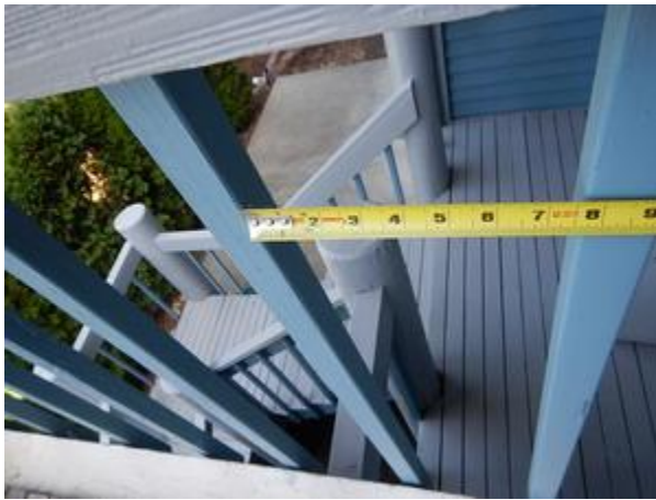
7+ inch baluster spacing
