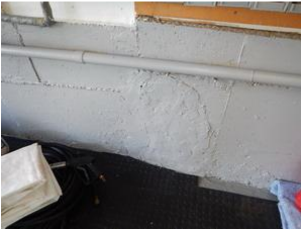
patch or repair to foundation wall
