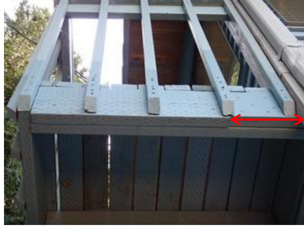
original supported joists carrying replacement components
