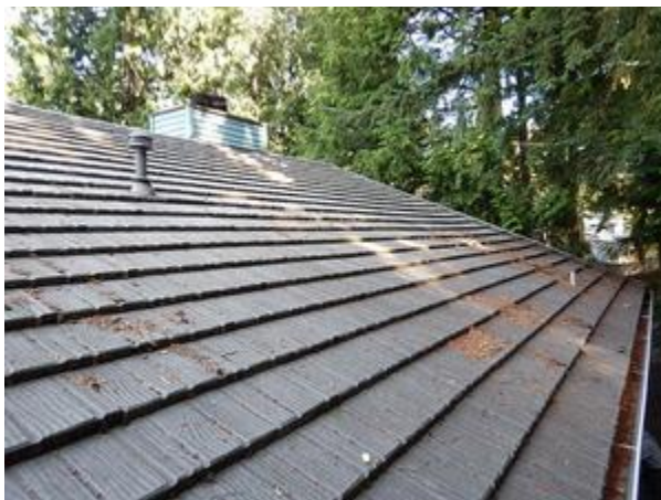
metal shingle roof, typical
