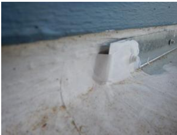
14 15 amateur flashing repair not watertight 16
