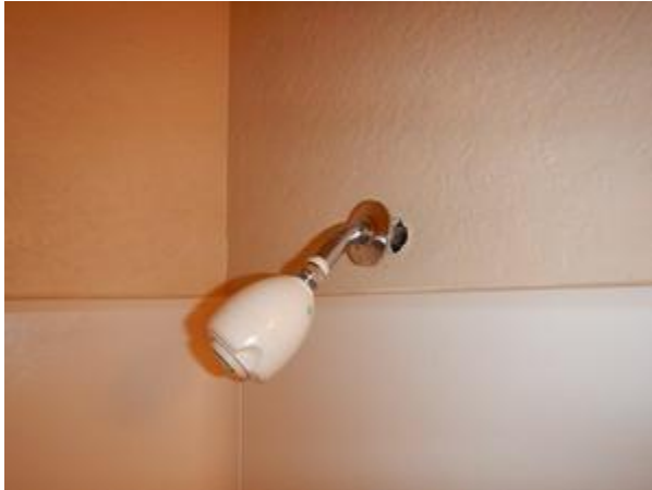
showerhead is not properly secured
