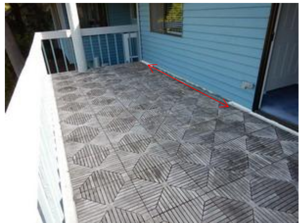
14 15 amateur flashing repair not watertight 16
