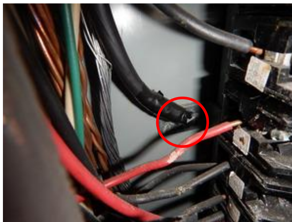
improperly terminated conductor
