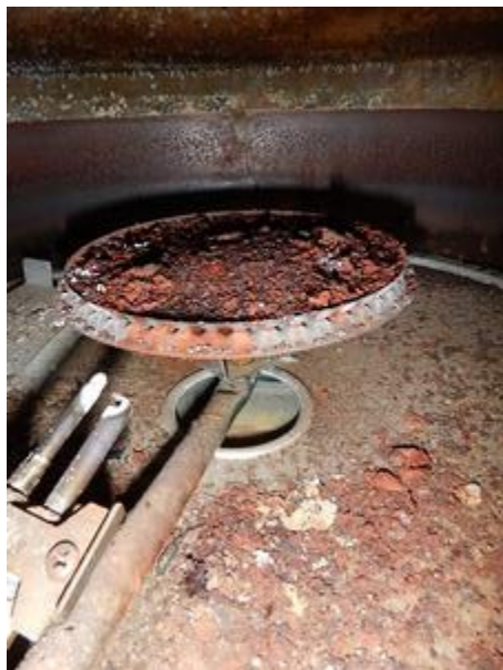
21 corroded turbulator debris on burner 22
