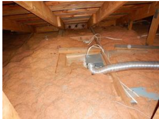
disturbed/missing insulation at retrofit fans
