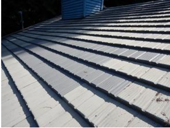
numerous shingles have been replaced
