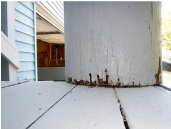
decay noted in all of the peeler poles
