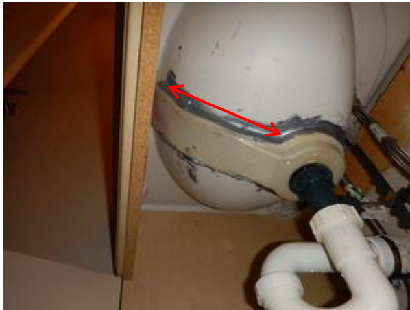
high volume leak in overflow channel
