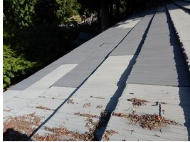
numerous shingles have been replaced
