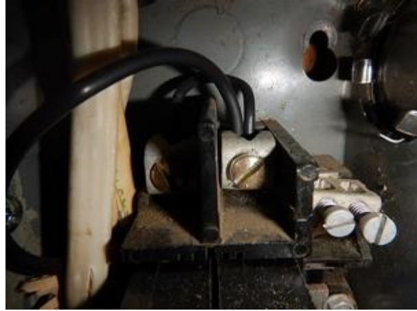
double tap in garage sub-panel
